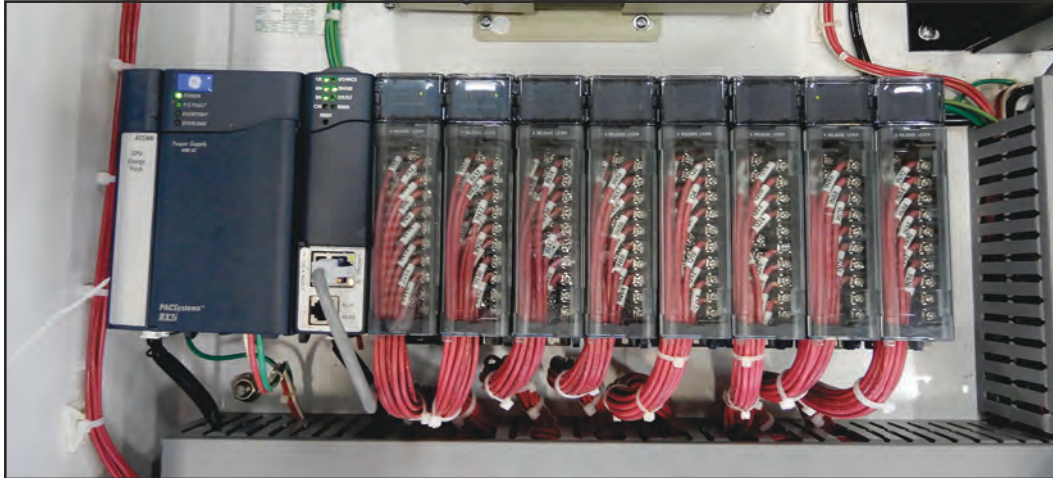
Figure 6-3: PLC in Main Electrical Enclosure
