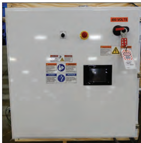
Figure 1-2: Sample of a Lockout/Tagout Mechanism on an Electrical Enclosure
