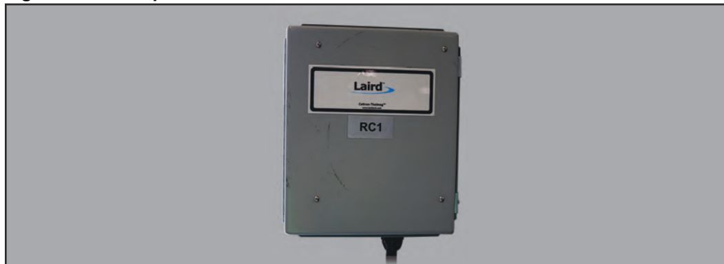
Figure 6-2: Example of Radio Controller Electrical Enclosure
